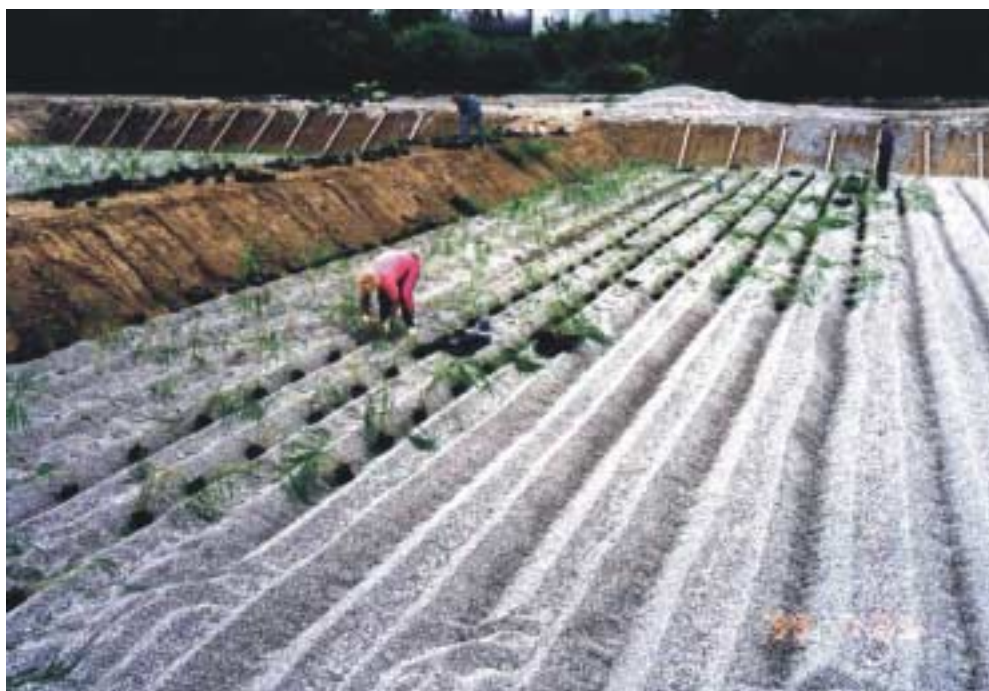
Figure- 8 Planting of potted seedlings in a sludge mineralization bed.
