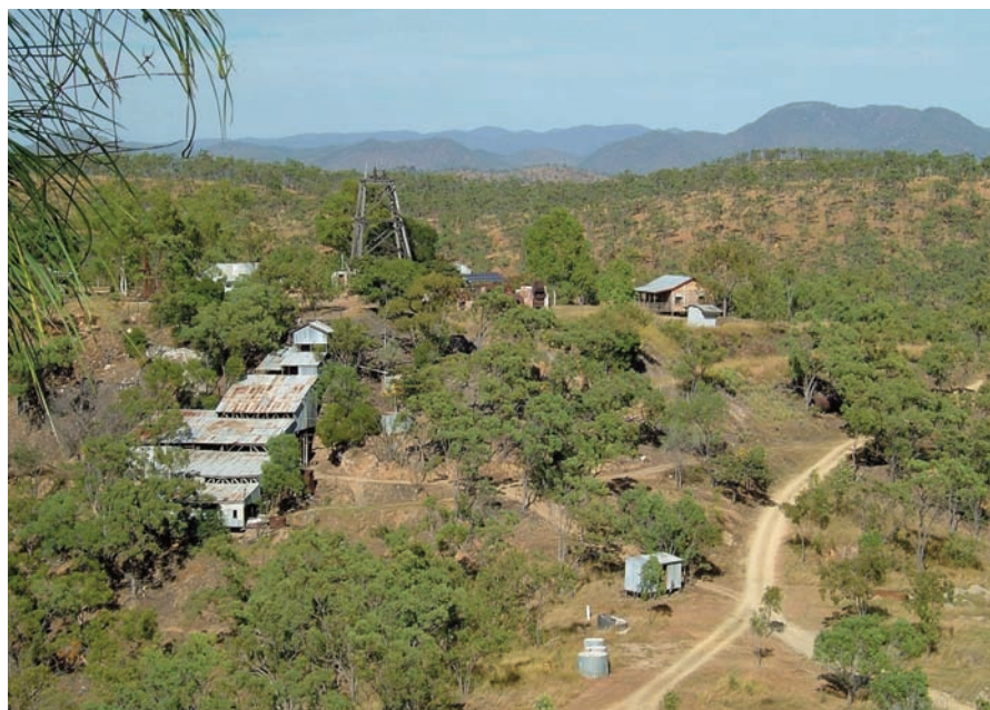
Fig. 1. Abandoned Tyrconel/Australia gold mine site. The headframe stands about the flooded main shaft.
