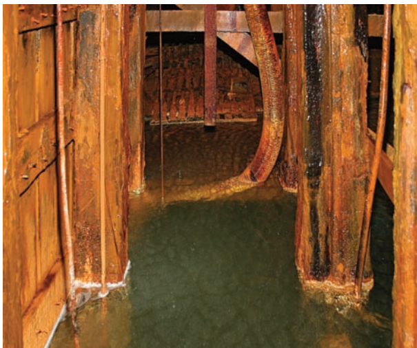
Fig. 15. The flooded Reiche Zeche shaft of the Freiberg/Saxony mining field (2 March 2006). The brown colour is a result of ochre precipitates as a consequence of the catastrophic flooding of August 2002. Width of picture approximately 2 m.
