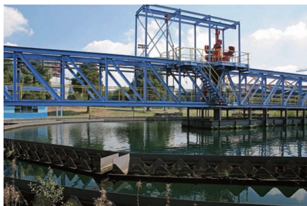
Fig. 88. Radial flow clarifier of an active mine water treatment plant at As Pontes lignite mine (Spain).
