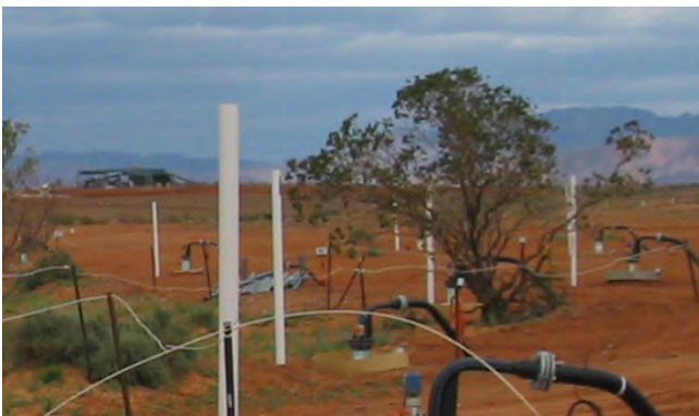
Fig. 2. Wellfield within an environmentally sensitive area (creek), where environmental impacts (surface disturbance) were minimized to preserve vegetation.
