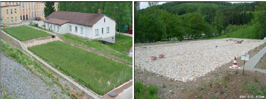
Fig. 8. Experimental multi-cell wetland at WISMUT's Schlema mine site (left: plant cells, right: microbiological cell with gravel bed).
