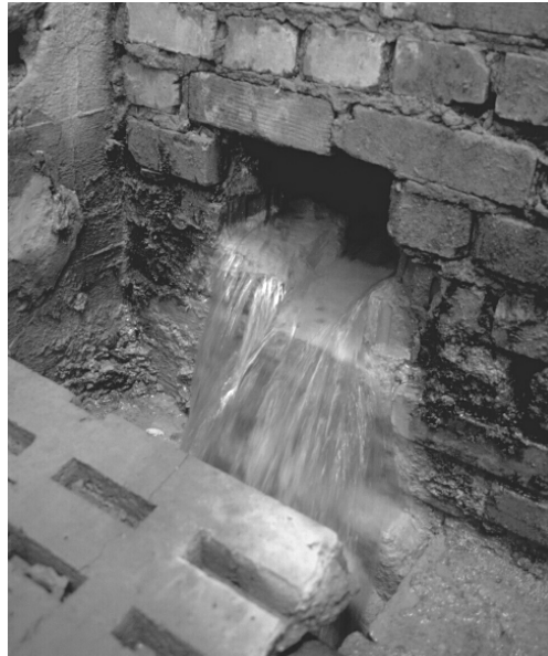
Fig. 4. Discharge point at the dewatering adit (MP1).
