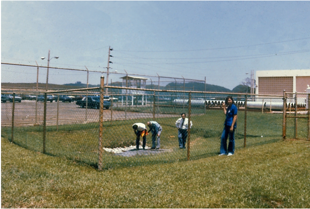
Figure 3. (Left) Restricted access to an improved sinkhole operating as a Class V injection well receiving treated industrial wastewaters at the RCA del Caribe facility, Barceloneta, P.R. (Right) Close-up view of sinkhole depicting concrete reinforcement for improvement of sinkhole sides, and wastewater-discharge pipe draining approximately 500 gpm of treated wastewater from the RCA facility. This Class V Well was operated under Permit No. 83-004 issued by the UIC Program under the authority of the Federal Safe Drinking Water Act; all facility operations at RCA del Caribe were ceased in 1987 (USEPA, 1994).
