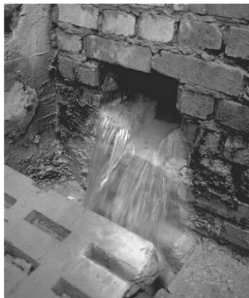
Figure 4: Discharge point at the dewatering adit (MP1).
