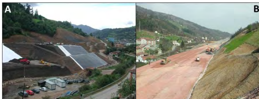
Figure 2. Mine waste encapsulation at El Terronal Hg mine (A), and road construction over encapsulated mine waste (B)
