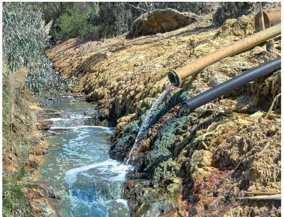
Figure 3 Contaminated water flowing from a pipe at the base of a tailings dam in the Witwatersrand
